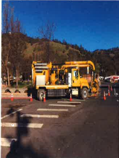
Jetting sewer line at plaza
