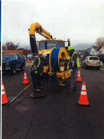
Jetting sewer line on Spinnaker
