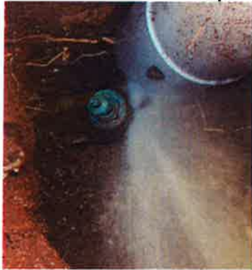
Before 2" main valve repair
