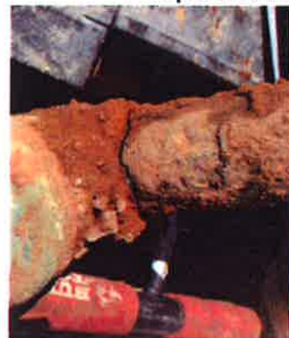
New 2" valve replacement
