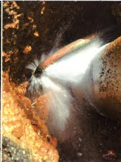
Leaking Saddle/ Main Repair
