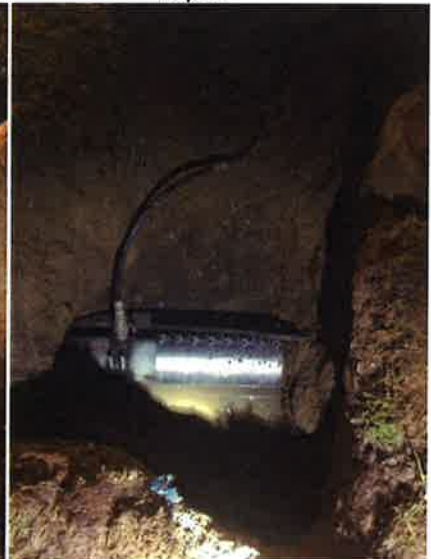
Main repair on Marina
