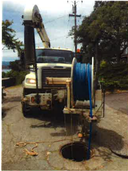
Jetting sewer line on Lakeview
