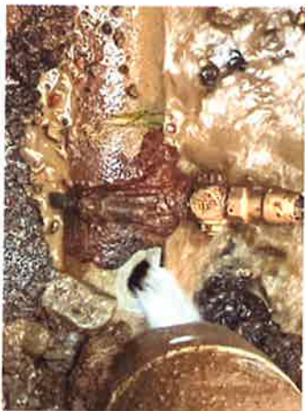
The bad saddle on hwy 20 4" main break on Short St.
