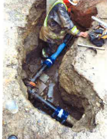
The bad saddle on hwy 20 4" main break on Short St.
