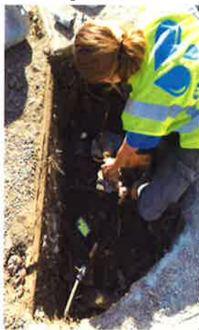
Installing New Service line
