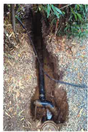
New Sewer lateral Shoreview
