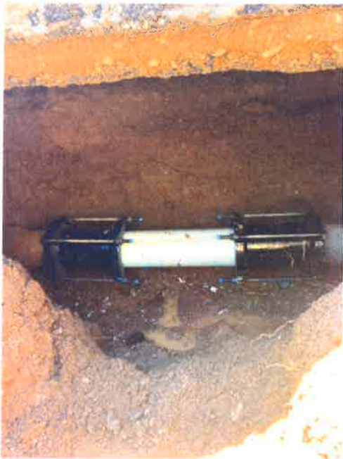
Replaced 36"x6" water main on Hwy Leaking service line on 6 th St
