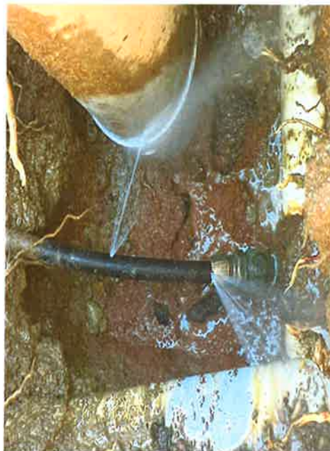
Replaced 36"x6" water main on Hwy Leaking service line on 6 th St
