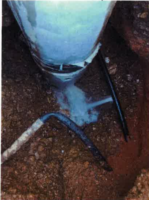
2 nd Street leak repair
