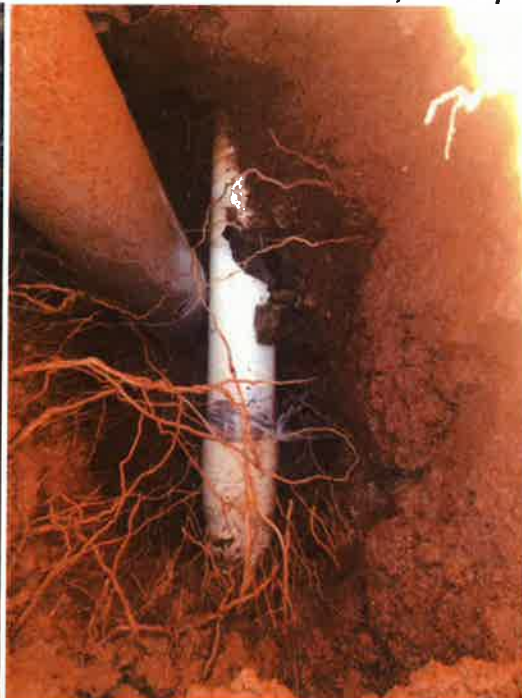
Lakeview bell cracked on main, leak repair
