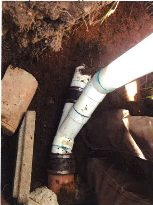
Replaced district approved clean out
