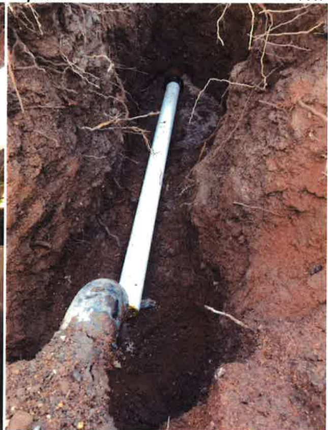
Replaced district lateral that was filled with roots
