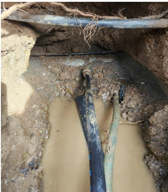
New 1” Service line
